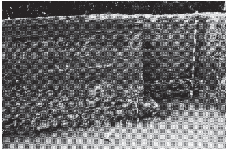
Fig. 3. The southeast corner of tower 1 and southern face of the North fortress wall (after VAGALINSKI 1999, 232, Abb. 4)
