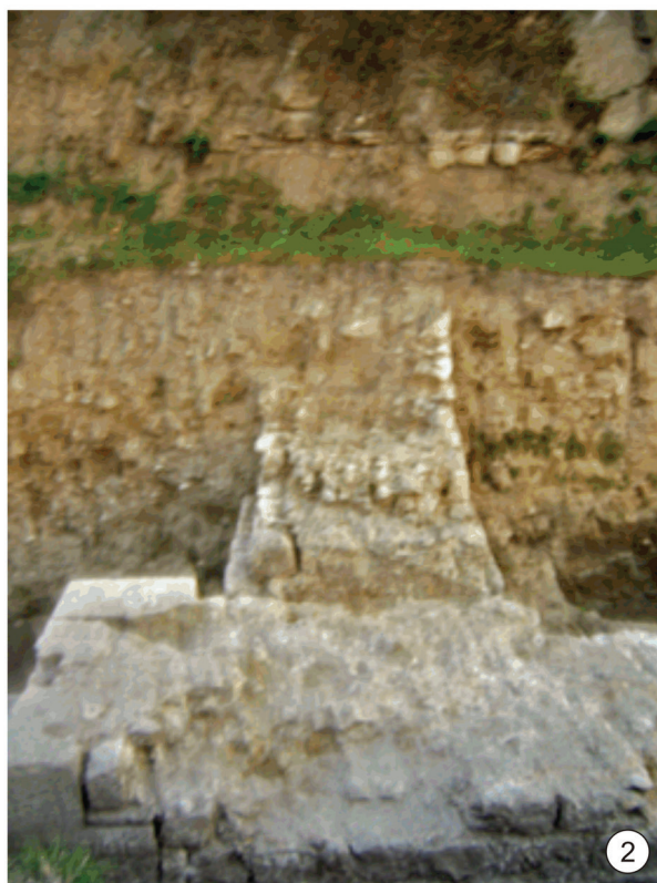
Fig. 8. Wall added to the North fortress wall: 1. View from the southeast; 2. View from the north (photos by Sergey Torbatov, 2010)
